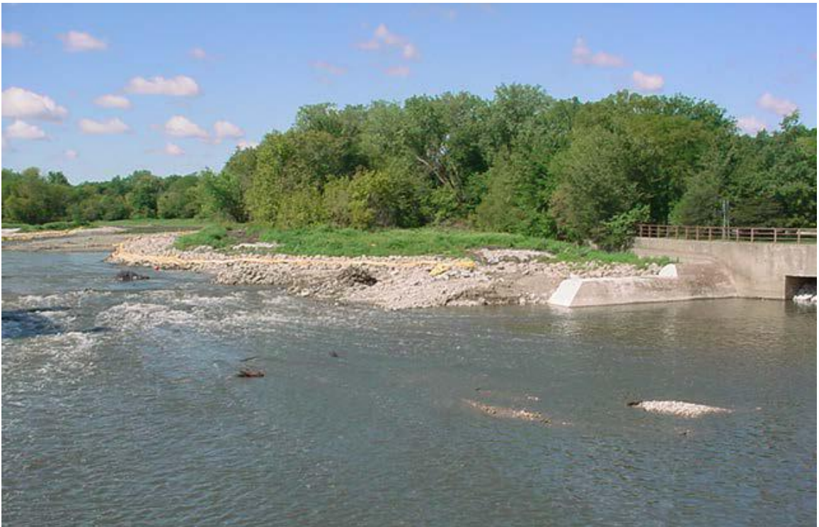
Figure 9: Removal of the Hofmann Dam with 30 foot long section remaining on left bank, looking upstream (IDNR)
