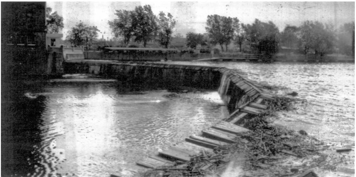
Figure 5: Horseshoe shaped Hofmann Dam constructed in 1908 with Hofmann Tower (IDNR)
